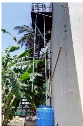
Image 8: Setup site in ICT Premises
